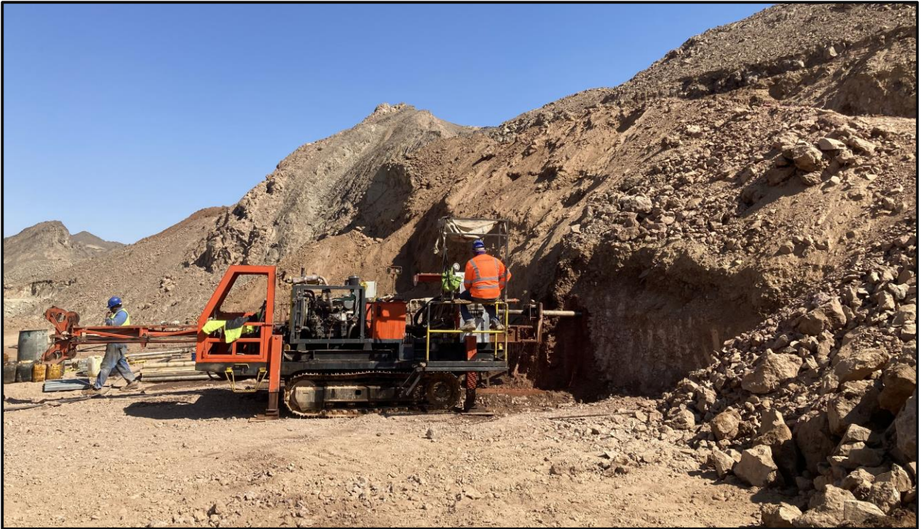
Figure 2: Energold's ID-500G rig drilling on hole HAD-020 at Hamama East
