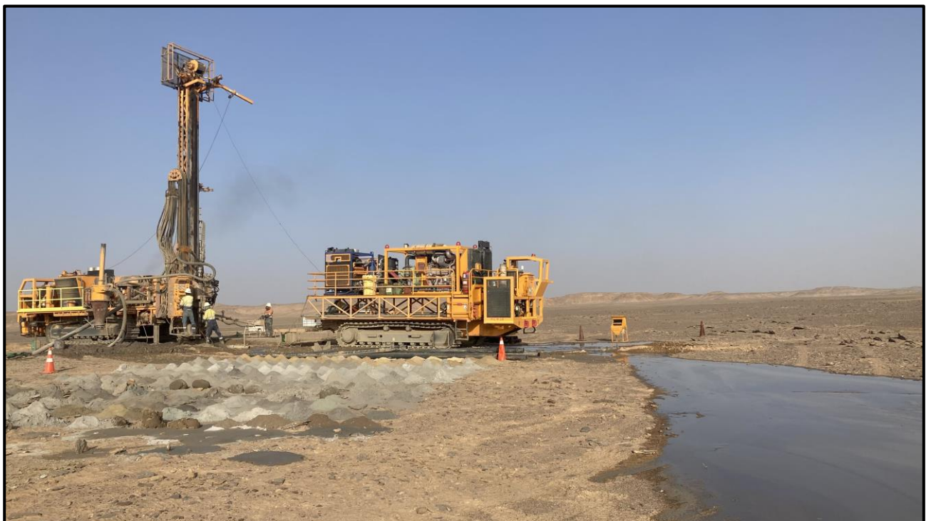
Figure 2: Drilling on groundwater exploration hole HAW-02
